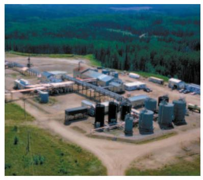
About 1 MBD of unconventional oil is currently extracted in Canada from facilities like this Steam Assisted Gravity Drainage oil sands facility. *Alberta, Canada*
