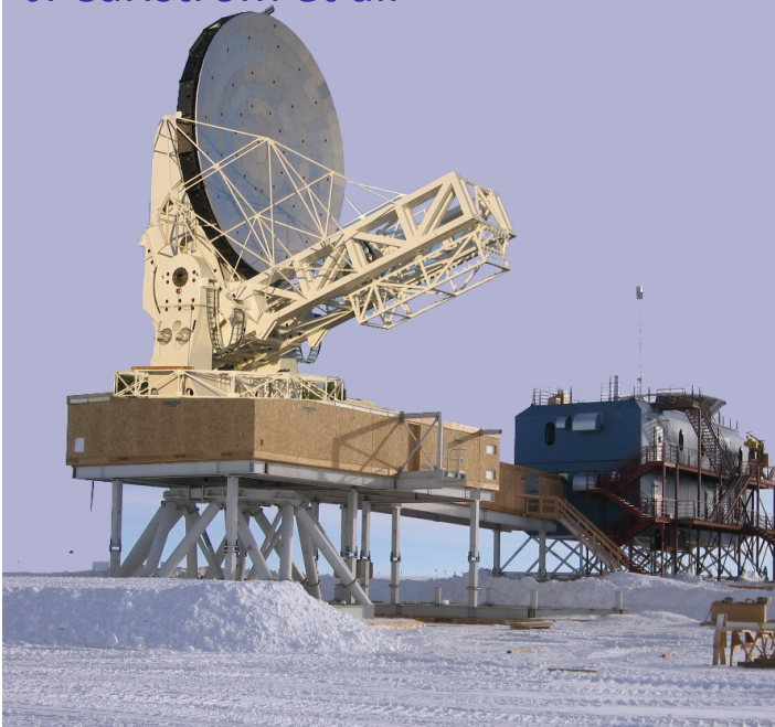
South Pole Telescope J. Carlstrom et al.
